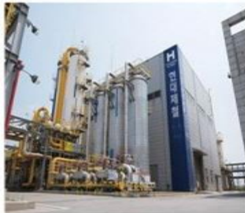
<Hydrogen Production Plant>
