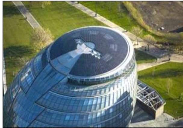
Solar PV acquisition (PV Installer)
